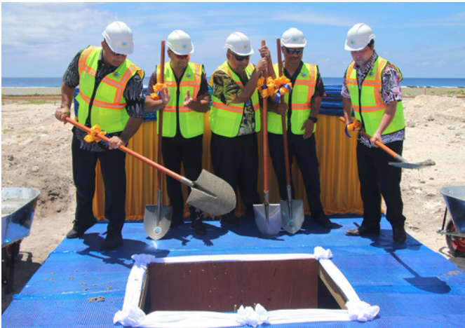
President Adeang pours first cement marking start of hotel construction
