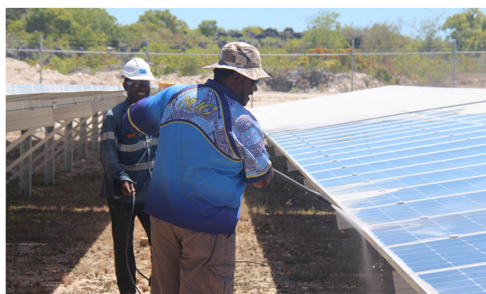
Nauru Utilities maintains the solar farm including regular wash-downs to ensure maximum solar absorption
