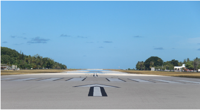
Resurfacing will extend life of runway another 20-plus years
